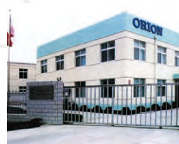
Shanghai Orion Chemical Co., Ltd. Shanghai I-Orion Machinery Co., Ltd.
